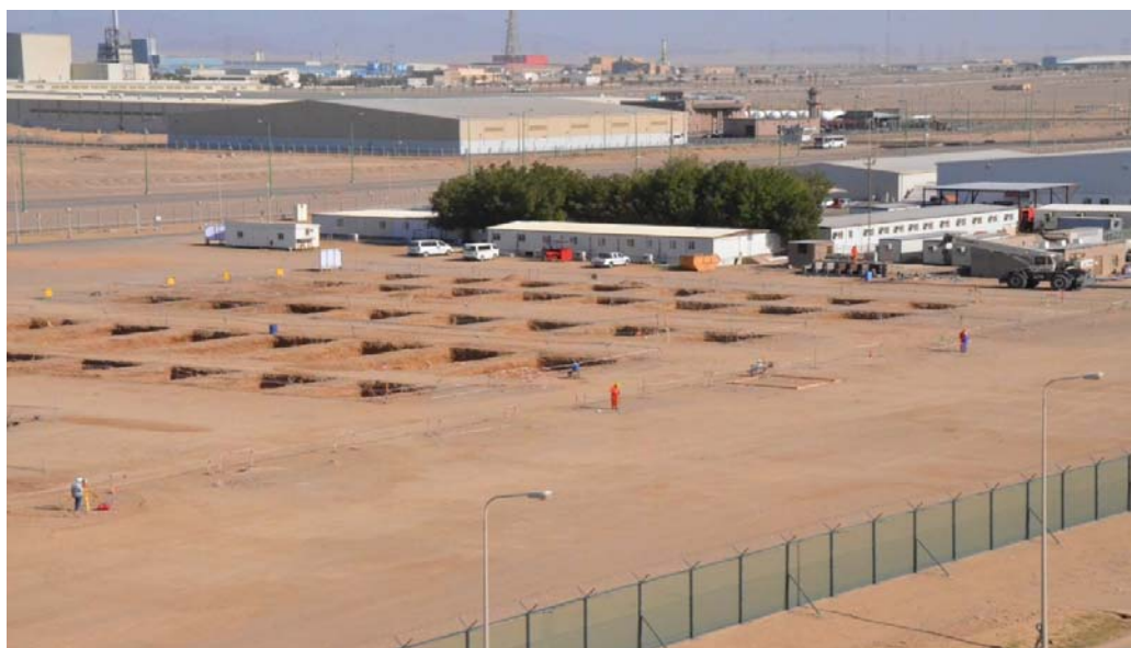
Natpet Schulman - Foundations Layout Plan
